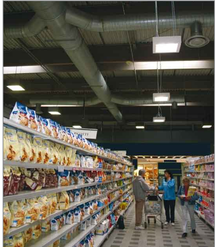
Today, LEDs allow even general lighting in supermarkets without compromising light quality.
