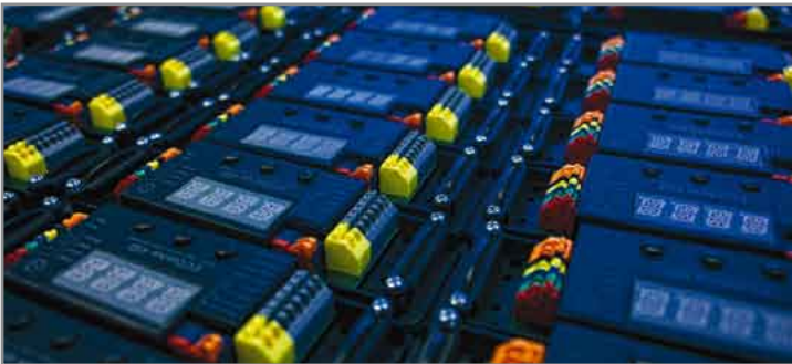
Figure 3: In DMX networks, RDM and LedSync provide a solution for many of these more intelligent network requirements: explore and address for setting up the network and temperature and other sensor feedback to the DMX controller can be implemented ensuring normal operational conditions prevail (Image: ©Fortunati 2009).
