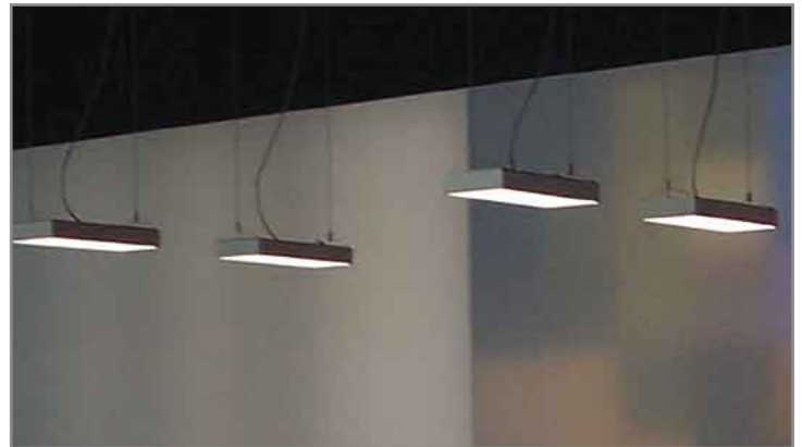
Figure 7: Pendant LED luminaires for office applications. Light is emitted by 11 high power LEDs and directed towards the work space by a microstructured optical cover. Glare reduction is also performed by the microstructure.
