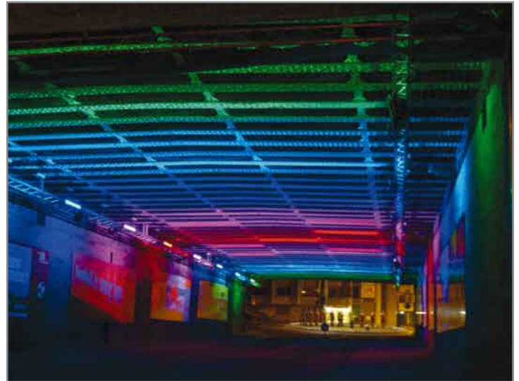
Figure 1: Passage to the Betzenberg, Kaiserslautern (Germany). RGB LED Lighting generates an attractive and inviting atmosphere and models the structure of the steel construction. (© Florian Schneider/Pixelio).
