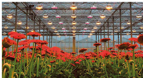
Plessey's new Hyperion high-power horticultural LED grow lights directly replace sodium lamps and cut energy by 40%
