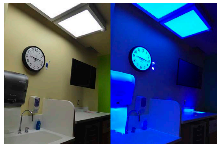
The research results from LRC showed the effectiveness of the tested system but it also suggests that UV-A resistant equipment and furnishing is required
