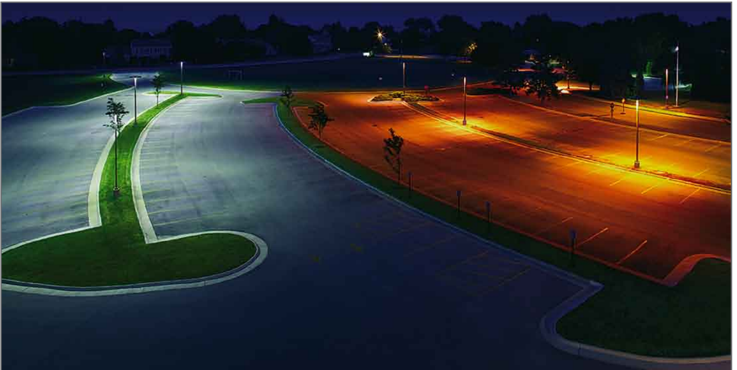
Figure 2: Parking lot with new LED lights (left) and original HPS lamps (right)
