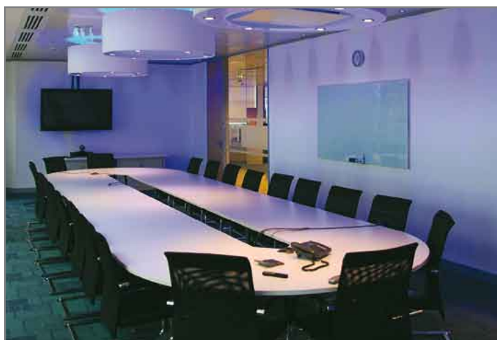
Figure 4: Meeting room entirely lit with solid-state fixtures
