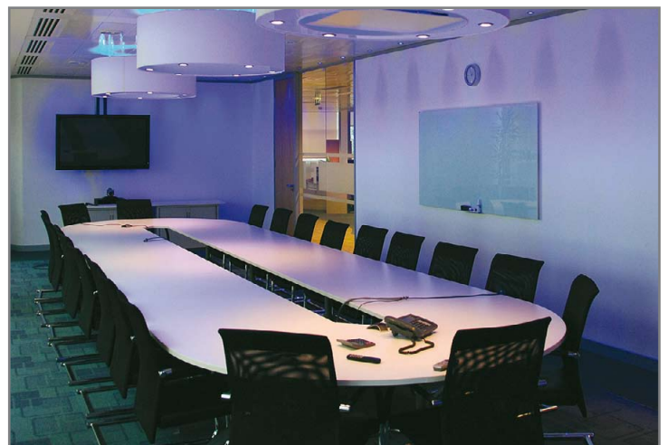
Figure 4: Meeting room entirely lit with solid-state fixtures
