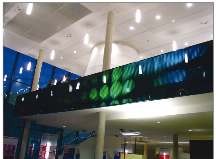
Figure 2: University of Darmstadt (Germany). The balustrade is covered by a 16 m wide RGB LED display to generate graphical effects and act as an info-board as well (© University of Darmstadt).
