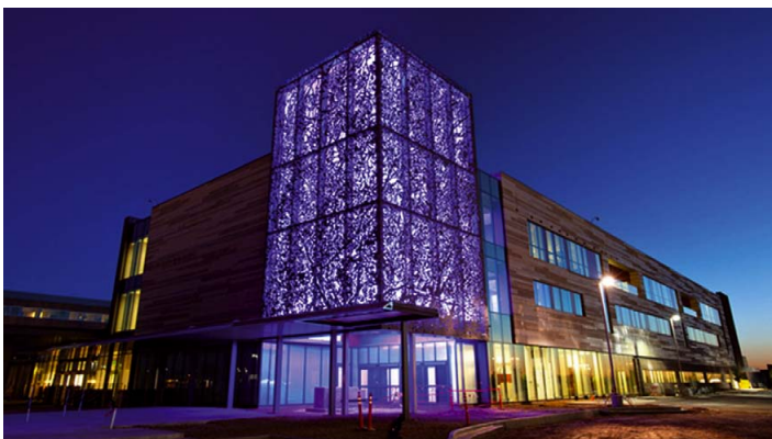
Lumenpulse transforms a tower into a beacon of light at night*
