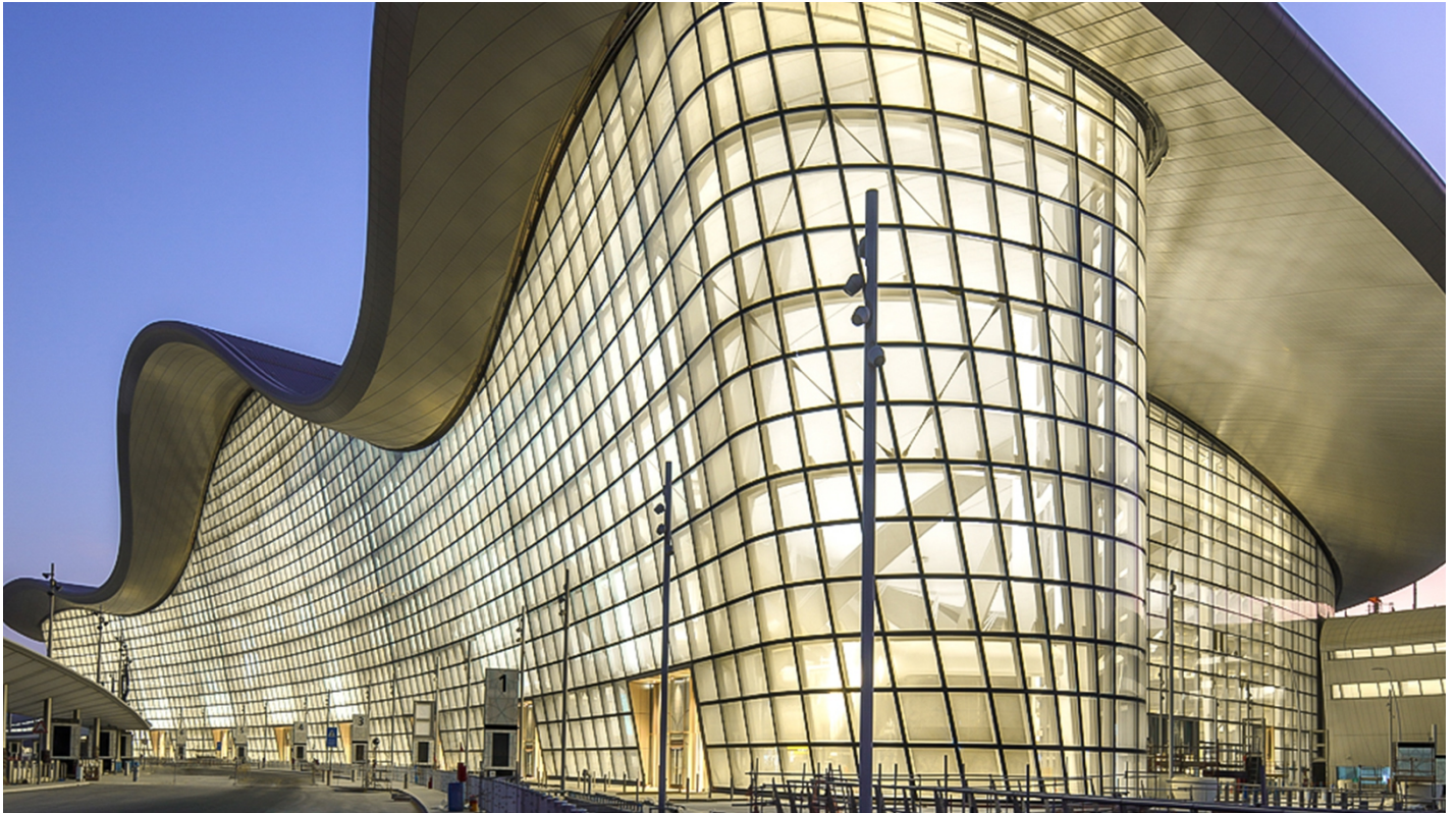
Delmatic's largest DALI control system in the world manages 235,000 normal and emergency luminaires throughout the 742,000 sq. terminal. The system seamlessly shares data with the building management, emergency power, fire safety, HVAC, AV and operational systems to maximize sustainability.
